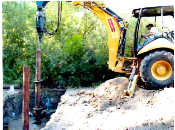
POSITIONING THE 8" CHPP
