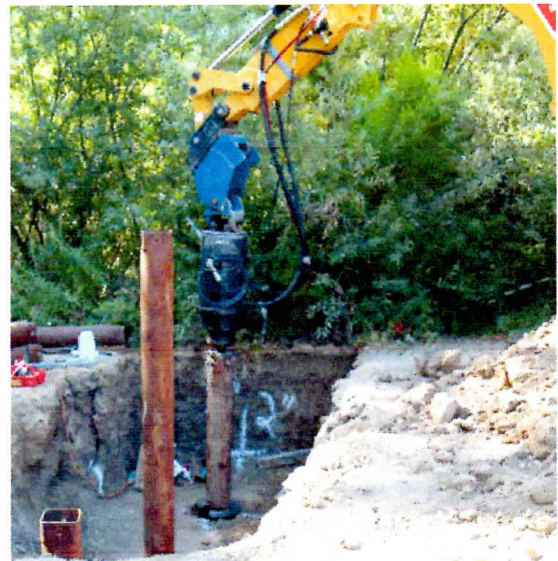
INSTALLATION OF THE 8" CHPP
