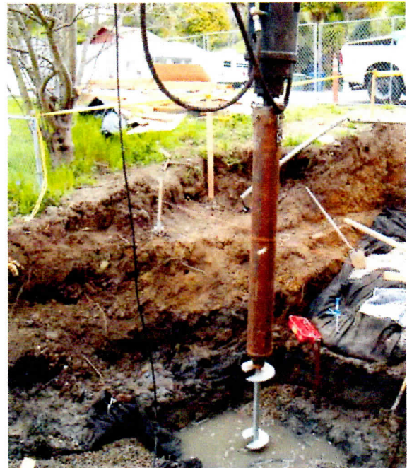
INSTALLATION OF THE 8" CHPP
